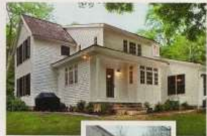
A better backyard to boot. The original two-story colonial had a shed-roof addition that created awkward massing between the two forms and a terribly boring back elevation. The new addition brings the forms together. The new rooflines and the window-seat bump-out add a lot of interest to enhance the colonial character.
